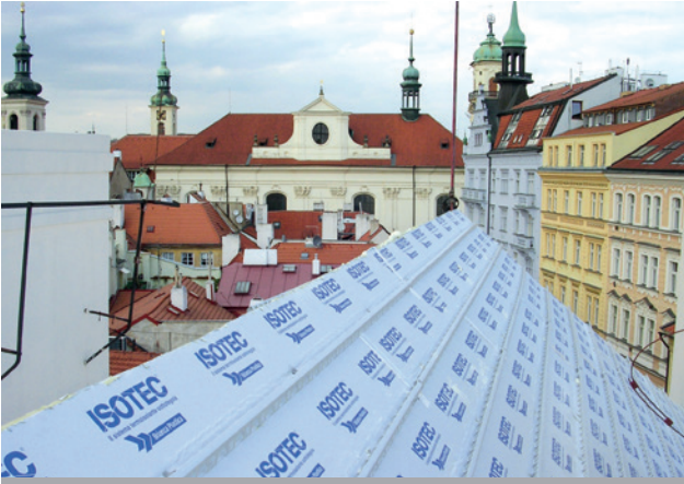
ISOTEC® - PITCHED ROOF IN PRAGUE OLD TOWN.
