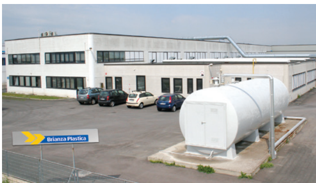
Brianza Plastica S.p.A. - Production site of Ostellato, Italy.
