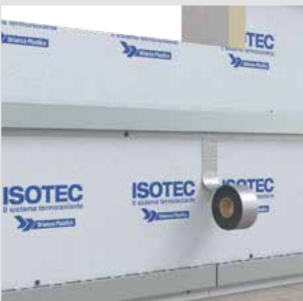
7 - Sealing of joints
