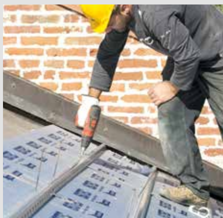
3- Positioning and fixing the panel
