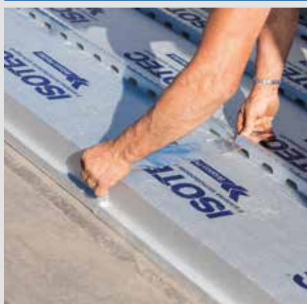
4- Applying butyl aluminium tape
