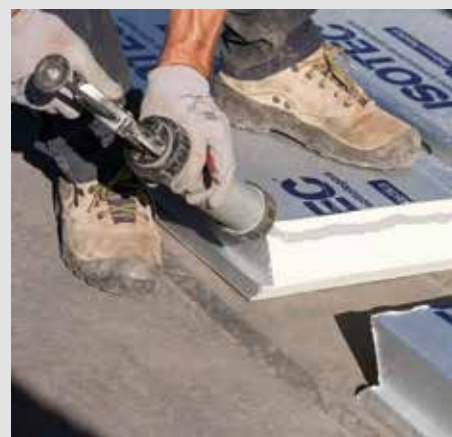
2- Sealing the dovetail with silicone
