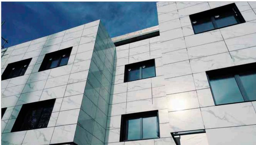
Isotec Parete has been fixed directly on the prefabricated infill panels in reinforced concrete. The 60 x 120 mm ceramic slabs have been anchored to the Isotec Parete steel stiffener by means of a special mechanical anchor in patented steel, which is inserted in the kerf cut on the thickness of the ceramic to create an attractive concealed effect. The final result is an **energy-efficient building of great appeal**, characterised by an original and elegant finish.
