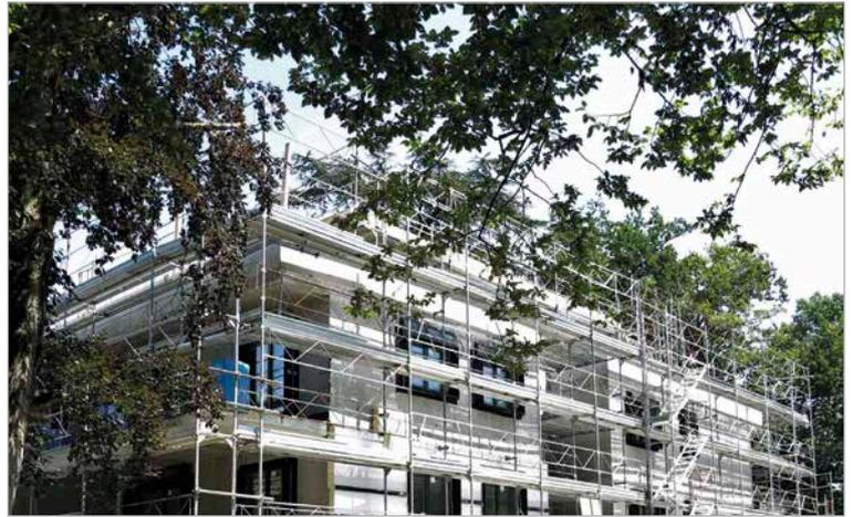
The structure of this new building, characterised by a geometric and linear architecture, is entirely in reinforced concrete and has been completely insulated with ventilated façades made of 160 mm thick Isotec Parete panels; for the external cladding has been chosen a ceramic white “Calacatta” marble glossy finish, for a very elegant effect, for a total surface area of 700 sqm.
